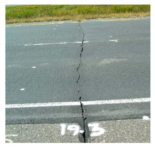
FIGURE 2 Reflected transverse crack through the slurry seal.
