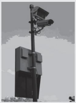
Rome's LTZ enforcement technologies include cameras that read vehicle number plates.
