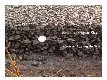
FIGURE 5-21 Example of a double-layer porous asphalt pavement used in the Netherlands. Source: Donavan (2006).
