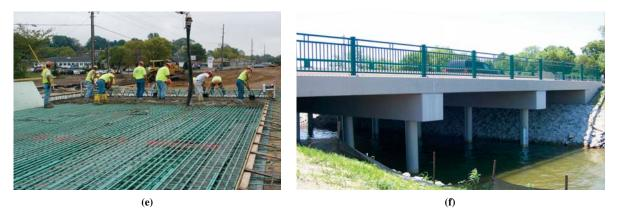
**Figure 1** Sequence of construction of a PCSSS: (a) precast pier caps in place, (b) Inverted T-sections in place (elevation view), (c) Inverted T-sections in place (plan view), (d) drop-in cage placed between precast webs for potential crack control, (e) deck reinforcement in place, and (f) finished structure.
