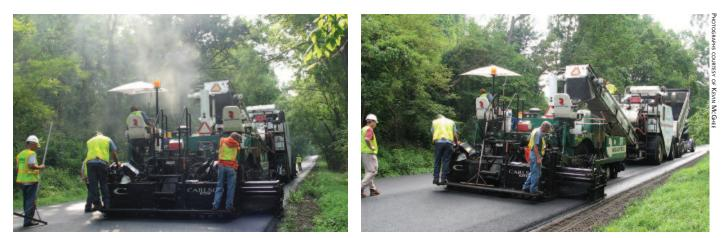
The reduction in visible fumes can be seen in a comparison of conventional HMA paving (*left*) and paving with WMA (*right*).
