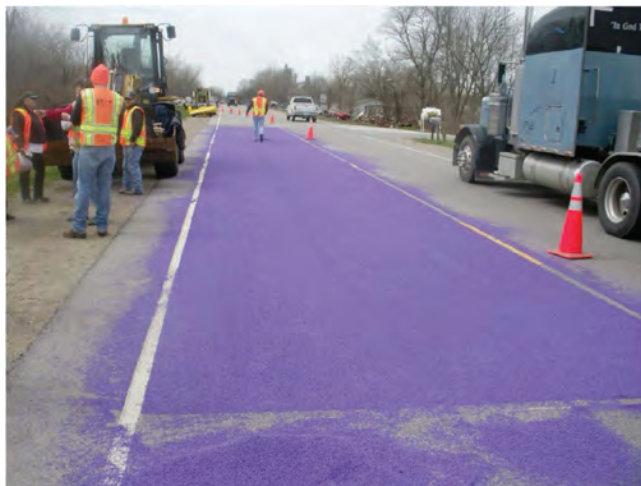
FIGURE 18 Colored pavement [Source: Russell and Godavarthy (2010)].
