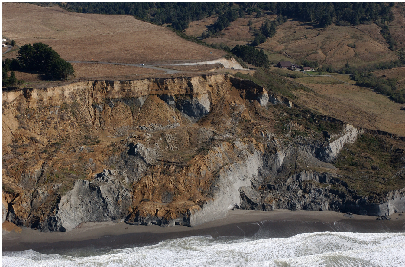
FIGURE 6.2 Large-scale landsliding along the Humboldt County, California, coast at Centerville. SOURCE: Copyright 2002–2012 Kenneth & Gabrielle Adelman, California Coastal Records Project, < www.Californiacoastline.org >.
