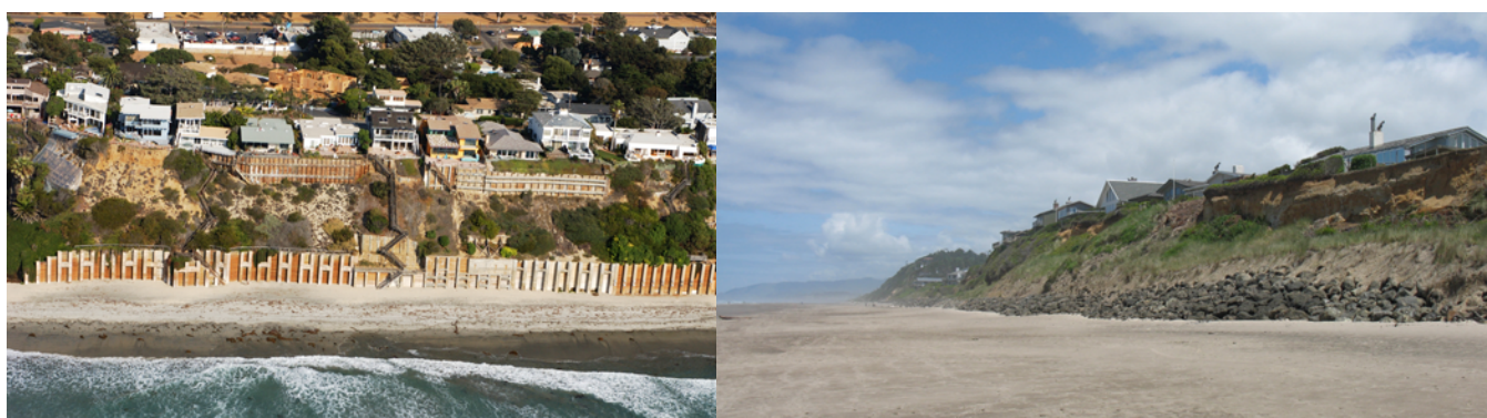
FIGURE 6.4 Seawalls and revetments fronting coastal cliffs and bluffs in California and Oregon. (Left) Concrete and timber seawalls protecting cliff top homes in Solana Beach, California. SOURCE: Copyright 2002–2012 Kenneth & Gabrielle Adelman, California Coastal Records Project, < www.Californiacoastline.org >. (Right) Rip rap protecting bluff top housing along the central Oregon coast. SOURCE: Courtesy of Gary Griggs, University of California, Santa Cruz.
