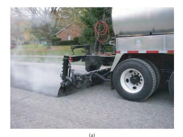
Figure 15. Uniform tack coat spray application.
