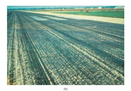
Figure 17 a, b. Non uniform tack coat spray application—improper nozzle setting.
