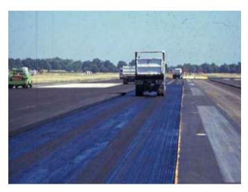
Figure 6. Pick-up by haul truck tires.
