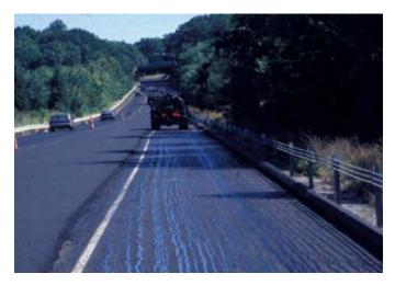
Figure 4. Non-uniform tack coat: streaks.
