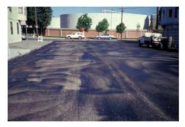
*Figure 13. Improper application of the tack coat using a hand wand.*
