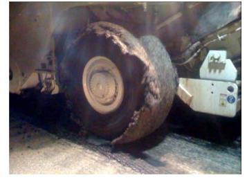
Figure 3. Tack coat and debris picked up by construction traffic from a dirty milled/tacked surface.
