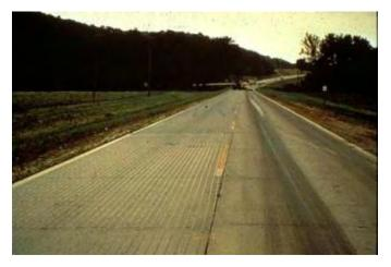
Figure 8. Poor spray pattern of tack coat due to improper nozzle alignment, nozzle size, and/or pump pressure.
