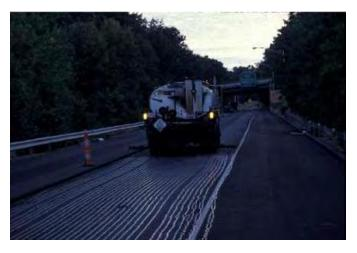
Figure 16. Non uniform tack coat spray application blocked and oversize nozzles.
