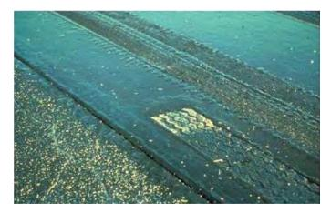
Figure 19. Excessive tack coat spray application.
