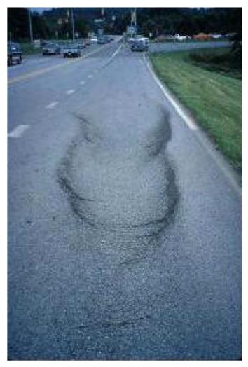
Figure 1. Delamination type of sliding failure.
