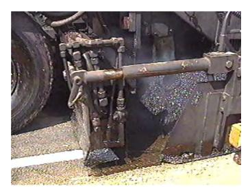
Figure 24. Tack coat application using spray paver.
