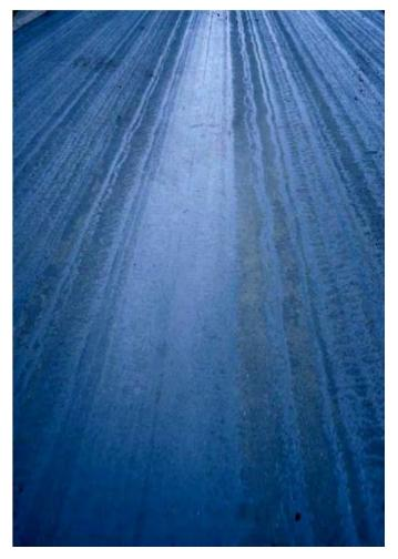
Figure 18. Non uniform tack coat spray application improper nozzle setting.
