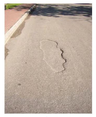
*Figure 25. Delamination failure in asphaltic concrete pavement.*
