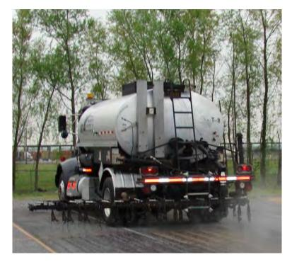
*Figure 15. Distributor truck spray application at 50% coverage.*
