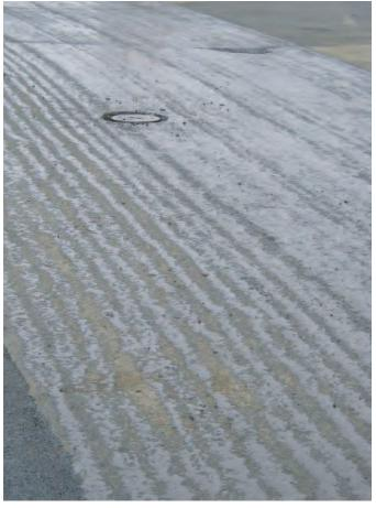
Figure 11. Tack coat spray applied with partially blocked nozzles.
