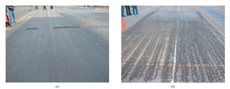
Figure 16. Tack coat application (a) 0.155 gal/yd<sup>2</sup> with 100% coverage and (b) 0.031 gal/yd<sup>2</sup> with 50% coverage (SS-1h).
