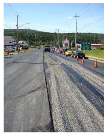
*Figure 22. Pick up of tack coat material by construction traffic.*
