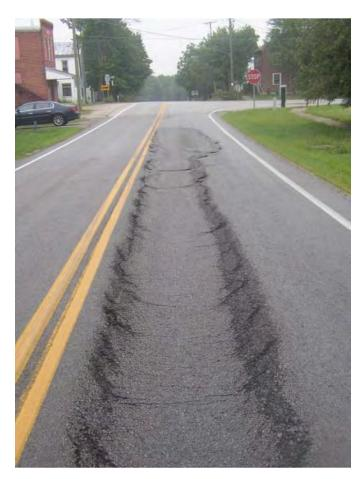
*Figure 26. Sliding failure in asphaltic concrete pavement.*
