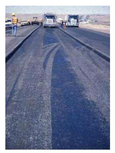
Figure 21. Pickup of tack coat material in wheel paths by construction traffic.
