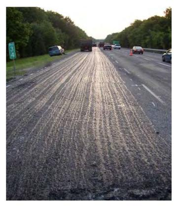
Figure 20. Non uniform tack coat spray application nozzles are not functioning and not at the correct angle.
