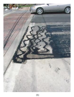
Figure 12. Improper application of tack coat using a crack sealing bucket.
