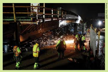
In early 2012, Utah DOT and contractor Provo River Constructors moved the Sam White Bridge using accelerated bridge construction techniques perfected through NCHRP research. The two-span bridge was the longest ever to be moved in the Western hemisphere.
