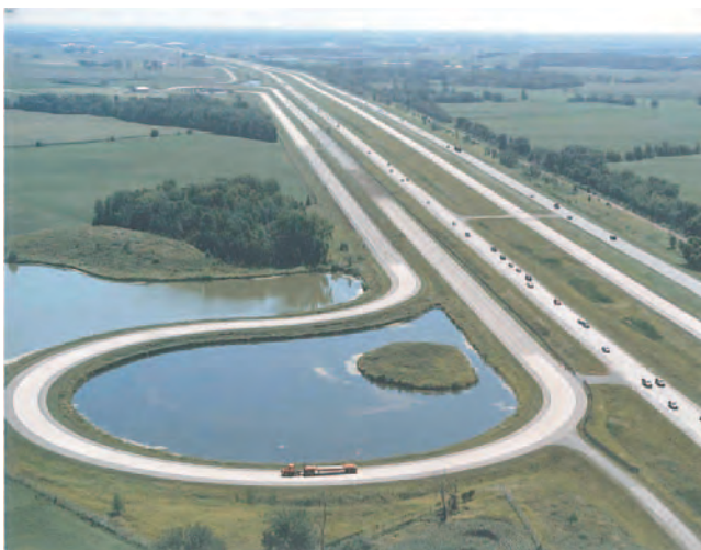
FIGURE 11 MnROAD test track.
