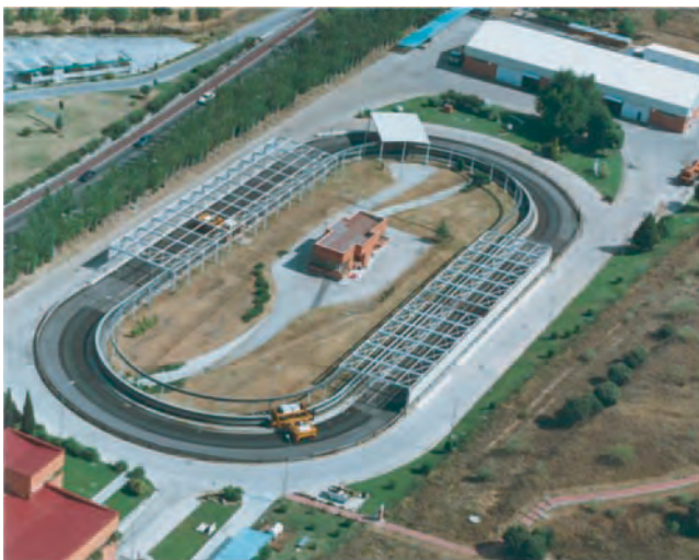
FIGURE 34 CEDEX f-sAPT facility.
