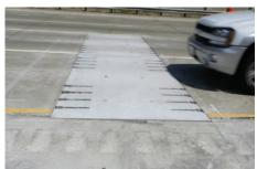
SAVING MONEY THROUGH RESEARCH— Working from SHRP 2 guides that comprise research results and extensive field testing to facilitate easier selection, design, fabrication, and installation of precast concrete products, the Illinois Tollway is using precast concrete pavement panels in a large road repair project. The Tollway reports that this decision will save at least \$500 per panel—in a project that involves placing more than 700 panels—compared to the typical method of full-depth replacement.
