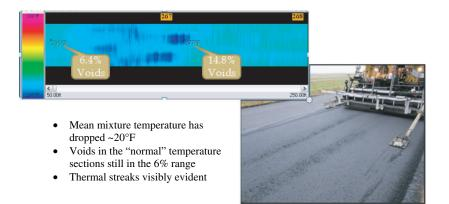
*Figure 3.61. Significant thermal segregation on Region 3 demonstration.*
