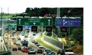
Figure 3.2. Variable speed limit (VSL) control in Stockholm, Sweden.
