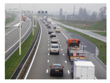
Figure 3.4. Implementation of plus lane (closed condition) in the Netherlands.
