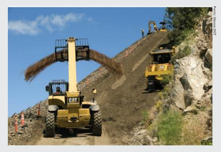
Contractors for Oregon DOT install rockfallmitigating wire mesh along U.S. 97 near Klamath Falls. The Rockfall Hazard System was developed in Oregon and now is used by more than 25 transportation agencies throughout North America.
