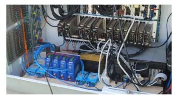
Figure 7.13. Optical sensors attached to load switches in the main signal cabinet.
