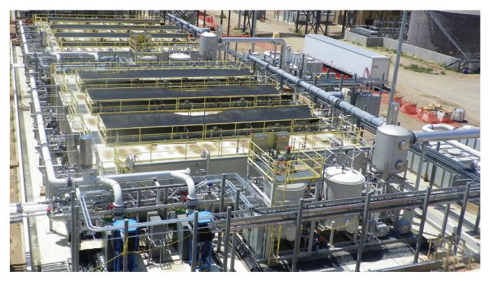
FIGURE 2-2 Two of the four biotreatment modules at PCAPP, each of which has four immobilized cell bioreactor units. SOURCE: Paul Usinowicz, Water/Wastewater Research Leader, Battelle, "Design and Operating Conditions for PCAPP's Biotreatment Process," presentation to the committee, November 28, 2012.
