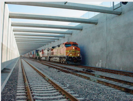
FIGURE A container train of the Alameda Corridor Freight Line in California. The trains travel in an open-braced trench that provides ventilation for the engines and grade separation for container traffic. SOURCE: Courtesy of the Alameda Corridor Transportation Authority
