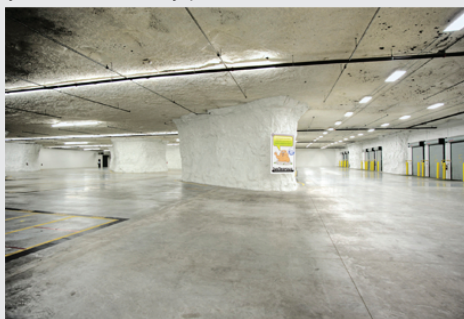
FIGURE Underground warehouse space in mined limestone caverns approximately 100 feet beneath Kansas. Roads and facilities can accommodate 18-wheeler traffic. SOURCE: Hunt Midwest, http://huntmidwest.com/press.html .
