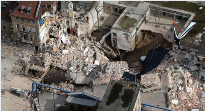
FIGURE 1 Collapse of multiple buildings resulting from excavation collapse. SOURCE: AP Images.
