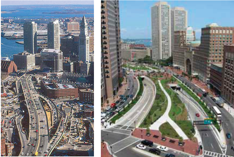
FIGURE 5.2 Boston Central Artery as an elevated structure and as an underground roadway SOURCE: MADOT, 2012.
