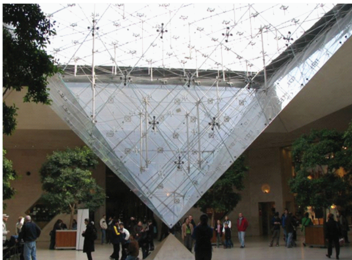
FIGURE 1.4 The inverted pyramid in the Carrousel du Louvre , an underground shopping mall in Paris, France, adjacent to the Louvre museum of fine art. The underground facility accommodates shopping, live theatre, auditorium space, parking, and underground access to the famous museum. The inverted pyramid is made of glass and allows natural light into the underground facility. SOURCE: Photo by Gard Karlsen, available at http://gardkarlsen.com .
