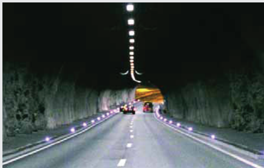
FIGURE 2 Some European tunnels use evenly distributed light-emitting diodes to help motorists discern the roadway edge and determine safe following distances.
