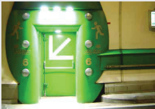
FIGURE 1 Example from Mont Blanc Tunnel (between France and Italy) of tunnel escape route signage, typical of the uniform signage used throughout many countries in Europe.
