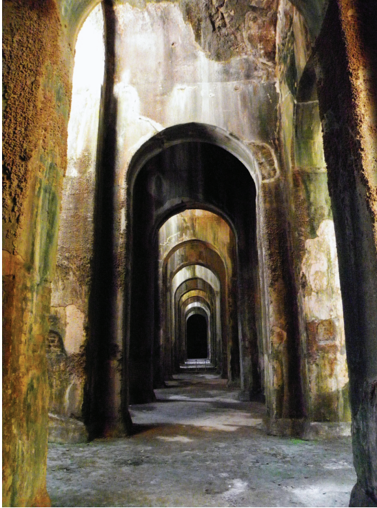
FIGURE 1.2 The Piscina Mirabilis in southern Italy was a 12,000 cubic meter capacity cistern carved by the ancient Romans between 33 and 12 B.C.E. SOURCE: Ra Boe/Wikipedia, License CC by-sa 3.0, available at http://en.wikipedia.org/wiki/File:Piscina_Mirabilis_2010-by-RaBoe-18.jpg .
