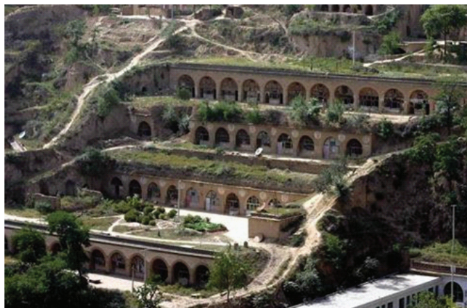
FIGURE 1.1 Example of a multistory yao dong , a type of cave dwelling carved into vertical or near vertical walls of loess (a silty soil), in the Shaanxi province in northwestern China. Approximately 90 percent of rural dwellers in the region lives in yao dong . SOURCE: Liu, 2009. License CC BY-NC-SA 3.0.
