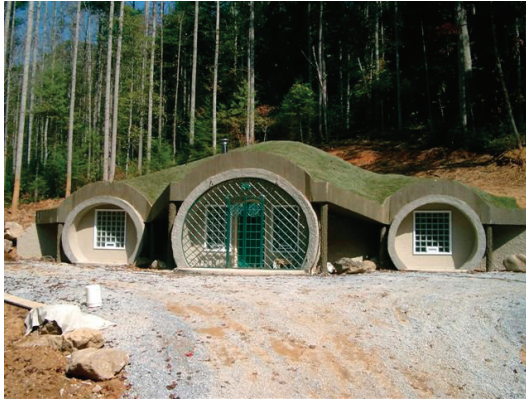
FIGURE 3.1 The earth-sheltered home is partially underground, providing greater strength and energy efficiency. SOURCE: http://www.monolithic.com .
