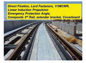
FIGURE 8 Direct fixation (DF) track.
