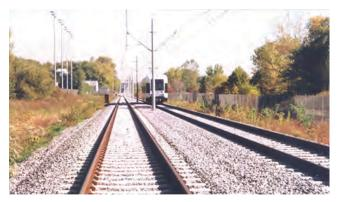
FIGURE 9 Ballasted track. Concrete ties, 115 rail, CWR, e-clip, with #3 ballast and overhead catenary.
