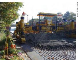
Construction of a concrete overlay on the E40/A10 road from Brussels to Ostend in Belgium. Preservation techniques to extend pavement service life are presented in the SHRP 2 Report Using the Existing Pavement In-Place and Achieving Long Life.
