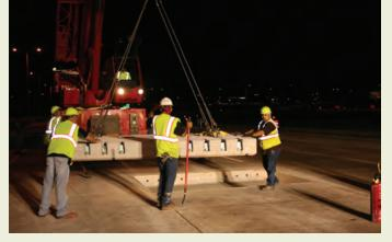
Crews place a precast panel on the central Tri-State Tollway, Interstate 294.
