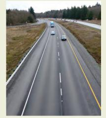
Old concrete panels beneath I-5 in Washington State caused severe cracking in the roadway (top). Washington State DOT piloted a webbased decision support tool for inplace pavement recycling and seated the concrete with an asphalt concrete overlay (bottom).
