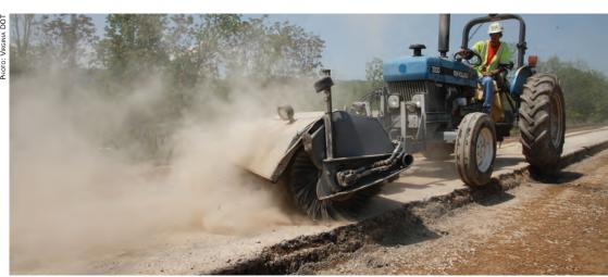
In-place recycling on I-81, a major thoroughfare in Virginia. Methods to incorporate in-use pavements into new, long-lasting pavement structures can lead to faster and more costeffective in-place pavements. **SHRP 2 RENEWAL FOCUS AREA**
