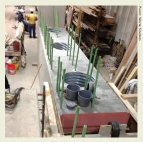
Vermont Agency of Transportation (VTrans) piloted techniques for precast bridge elements, such as this integral abutment, designed by a VTrans team.
