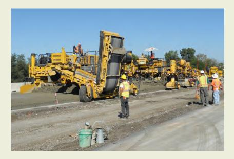
A two-lane belt placer spreads the top lift of concrete over a bottom lift of "green" concrete in front of a slip-form paver, creating a composite pavement on the Reagan Memorial Tollway.
