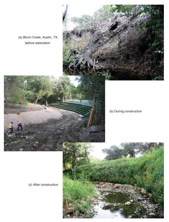
*Figure 1.3.* Typical biotechnical river restoration project protecting an eroding bendway (photo courtesy of City of Austin, TX, Watershed Protection Department).
