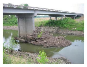
*Figure 1.1.* Drift accumulation on a single bridge pier (photo courtesy of Ayres Associates).
