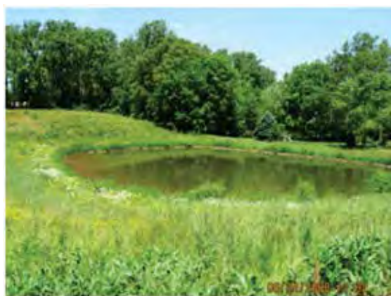
FIGURE 12 Wet retention pond. (Photo: http://rwmwd.org/ ).
