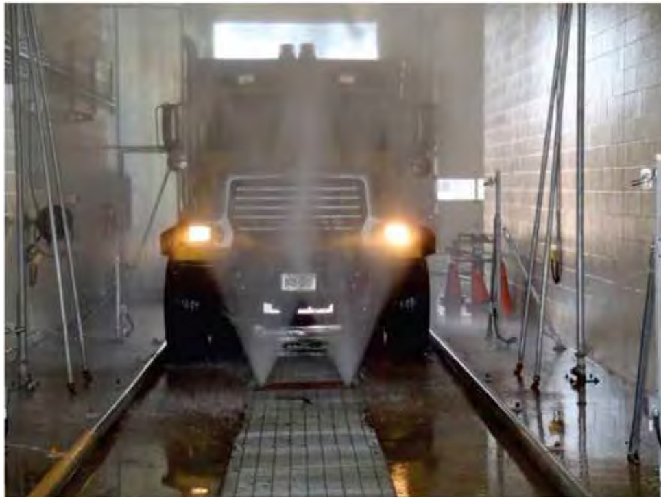
FIGURE B4 A tandem-axle salt truck being washed off following a salt spreading operation. Washwater is then collected through the grates in the floor and stored in underground tanks in the washbay. From that point, the recycled wash water can be pumped through the brine machine and stored as salt brine or be blended with an alternative product (Courtesy: City of Toronto).
