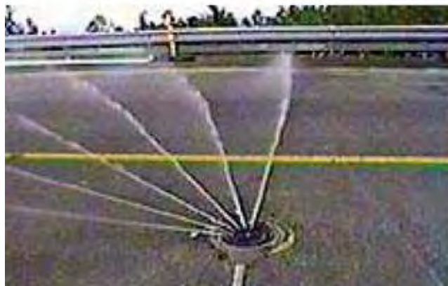
FIGURE 16 A FAST system on a bridge in action (Pinet et al. 2001).
