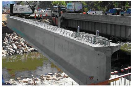
Bridge girders over the Weber River for the Utah I-15 NOW project, which relied on a design–build delivery method for completion in time for the 2002 Winter Olympics in Salt Lake City.
