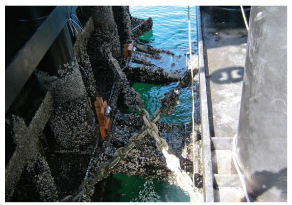
Ferry berth at Seattle, Washington, terminal, with linear motion transducers—cylindrical in shape—installed on the piers, just above the surface. Distance sensor installation at Auke Bay.
