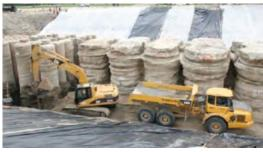
The contractor for the Tuttle Creek Dam Safety Assurance Project invented a new method of jet grouting; (above:) samples produced by the contractor for testing during construction.
