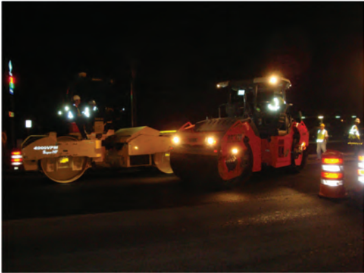
Intelligent compaction density evaluation in Utah.
