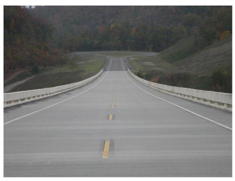
Figure 22. Primary sag vertical curve on the Smart Road.
