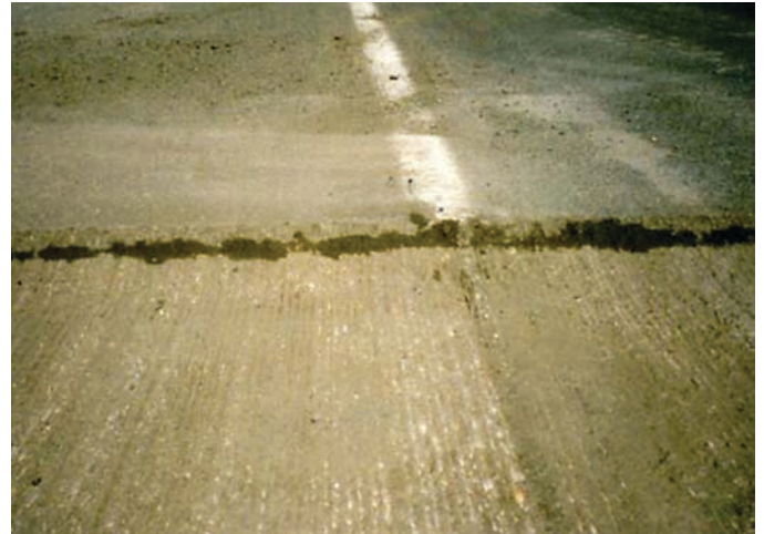
Figure 1.3. Moisture present at HMA layers interface.
