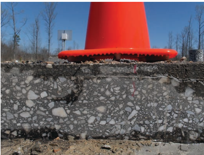
Figure 1.2. Delamination in an HMA pavement.
