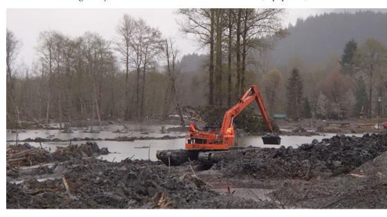
Amphibious excavator constructs a pilot channel to increase flow through the debris dam. the removal of the debris and to improve accessibility for the search and recovery operations.
