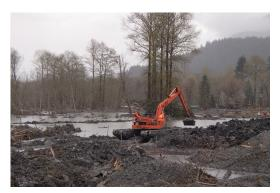
Amphibious excavator constructing a pilot channel to increase flow through the debris dam after the March 22, 2014, landslide—the deadliest in U.S. history—near Oso in northwestern Washington State.
