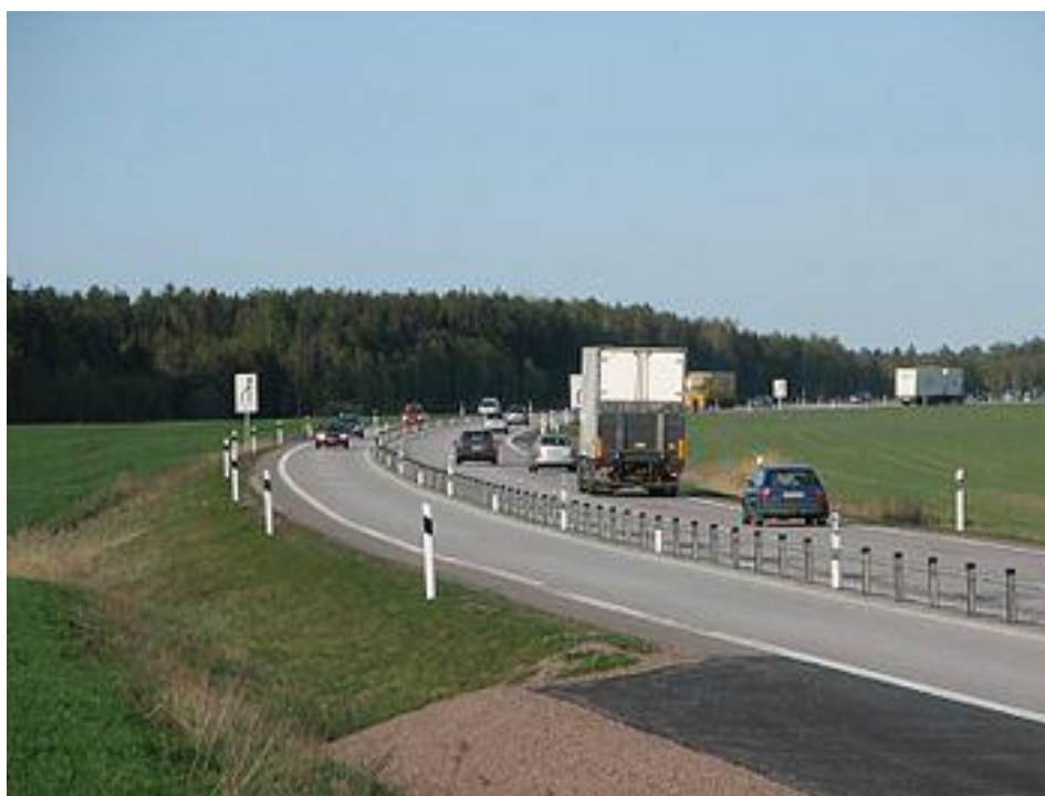
Figure 6.7. Example of movable cable median barrier.
