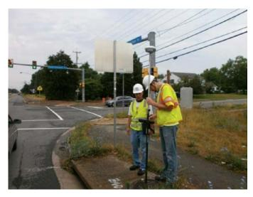
Figure 3.93. Establishment of survey control before geophysical investigations during in-service testing.
