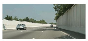
Figure 55. Highway with parallel noise barriers on opposite sides of the road.<sup>58</sup>
