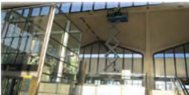
Electricians working on Terminal B cans
