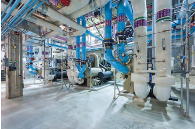
FIGURE 17 New power plant.
