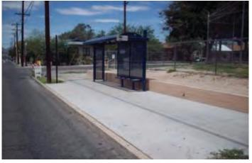
After: Improved bus stop with level lift area, accessible curb cuts and extended concrete pad allowing passengers to safely alight from rear of bus onto level surface with stable footing.
