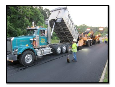
Figure 3.1. Paving operation on US-29.
