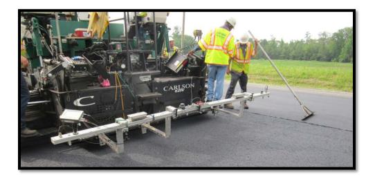
Figure ES.1. Pave-IR collecting thermal profile.
