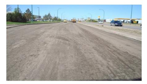
Figure B.4. Finished compaction of SS-1 emulsion stabilized RAP black base.
