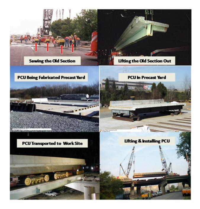
Figure B.33. Demolition–construction sequence (3).
