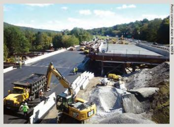
By eliminating the need for temporary roadways, the use of ABC techniques on the I-84 bridge in New York also reduced harmful environmental effects from the construction project.
