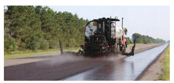
Fog sealing of a chip seal placed on state road.
