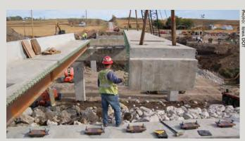
Precast bridge panels are installed on the US-6 bridge over Keg Creek Road in Iowa.
