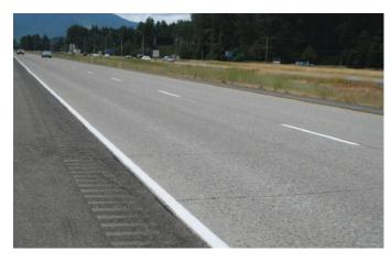
Figure ES.1. Photo of 35-year-old unbonded PCC overlay on I-90.
