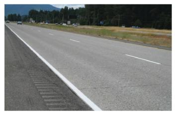
Figure 3.3. Photo of 35-year-old unbonded PCC overlay on I-90 MP 74.
