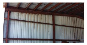
Figure 4.2. Rusted hangar not usable for aircraft storage. Source: Delta Airport Consultants, Inc.
