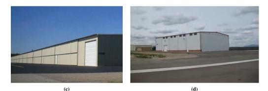
*Figure 3.8.* Hangar types: (a) shade, (b) T with simple door, (c) T with bi-fold door, and (d) box. Source: Delta Airport Consultants, Inc.
