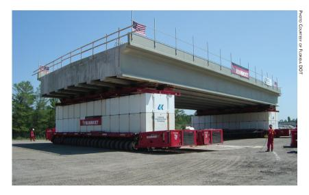
Self-propelled modular transporters move a bridge span into place within minutes. The results of research achieve value through use, by saving costs, time, and resources.
