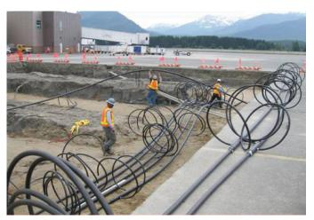
Installation of ground loop components of geothermal system at Juneau International Airport; City of Juneau.
