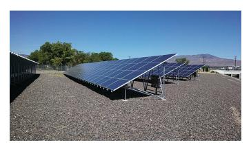
Figure 3-3. Fixed ground-mounted solar PV requires little O&M (Reno Airport ARFF building).
