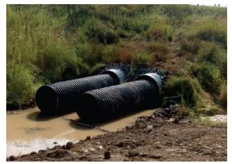
FIGURE 29 Sliplining 20-year-old corrugated steel pipe culverts with profile wall HDPE pipe. The annular space is filled with cellular foamed grout with specified strength of 210 psi (Doherty and Angelo 2012).
