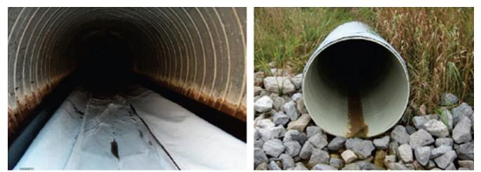
FIGURE 32 Cured-in-place pipe liner being installed and after installation in a 20-year-old corrugated steel pipe; 75-year service life assumed in design (Doherty and Angelo 2012).
