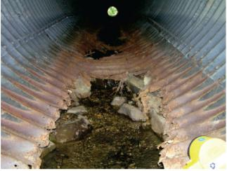
FIGURE 10 Corrosion accelerated by abrasion causing void formation below (Caltrans 2013).
