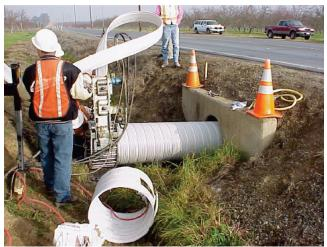
FIGURE 30 Expandable-diameter or spirally wound pipe liner being installed (Caltrans 2013).
