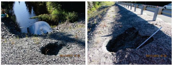
FIGURE 38 Failure of road embankment slope above a 12-ft-diameter structural plate corrugated steel culvert that had been extended at both ends. Perforation along bolt lines and 18-in. deflection at obvert of pipe.
