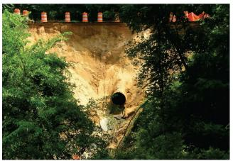
FIGURE 17 End treatment and scour failure at culvert outlet.
