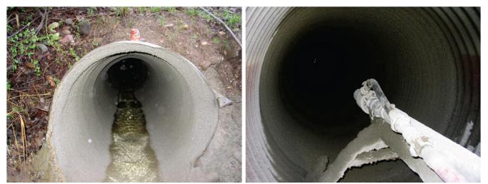
FIGURE 31 Examples of completed CSC liners (Source: Shotcrete Technologies Inc.).
