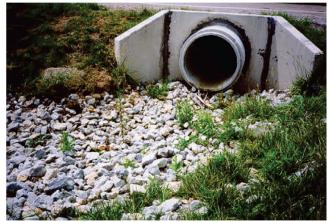
FIGURE 16 Example of outlet scour protection rock (*Source*: Ohio DOT).
