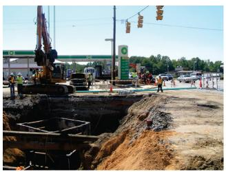
FIGURE 37 Emergency repairs following collapse of 30-in.diameter culvert near busy intersection.
