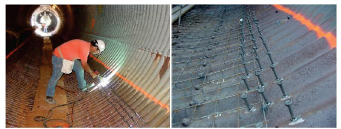
FIGURE 27 Shear connector welding studs (Nelson Studs) and wire fabric being installed prior to concrete invert paving (Caltrans 2013).
