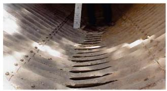
FIGURE 23 Perforated invert of metal culvert (Caltrans 2013).
