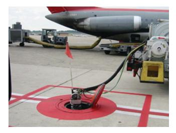
FIGURE 29 Marking and flag identification of fuel hydrant pit. (*Courtesy:* FAA.)
