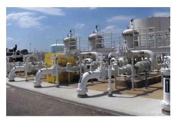
FIGURE 12 Example of parallel pumps for hydrant fuel system. (*Courtesy*: S. Quilty, SMQ Airport Services.)
