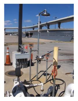
FIGURE 24 Example of eye wash and water deluge system at a fuel loading area. (*Courtesy:* SMQ Airport Services.)
