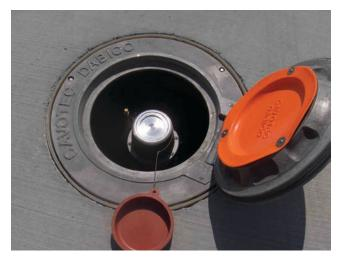
FIGURE 9 Example of a hydrant pit connection on a terminal ramp. (*Courtesy*: S. Quilty, SMQ Airport Services.)
