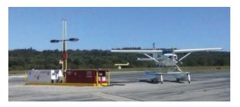
FIGURE 14 Typical fuel island arrangement with low-profile cabinets. (*Courtesy*: R. Lanman, Auburn–Lewiston Airport, Maine.)
