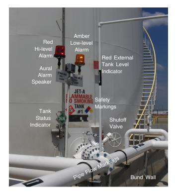
FIGURE 16 Example of a fuel tank's high-level and low-level alarms and markings. (*Courtesy*: S. Quilty, SMQ Airport Services.)
