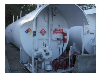
FIGURE 5 Example of a modular fuel tank. (*Courtesy*: S. Quilty, SMQ Airport Services.)
