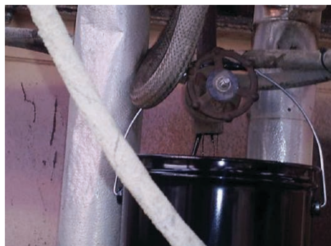
Figure 4-19. Foamed binder flow from sampling port, Plant 1, Cincinnati, Ohio.
