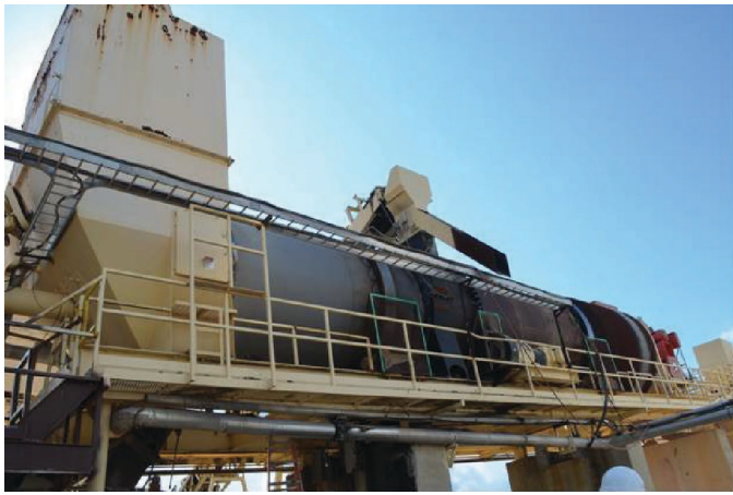
Figure 4-1. Counterflow drum plant, Austin, Texas.
