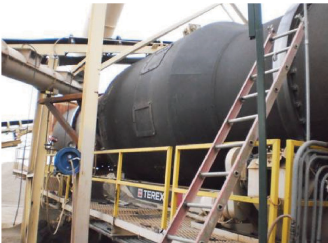
Figure 4-21. Terex counterflow drum, Plant 2, Fairborn, Ohio.
