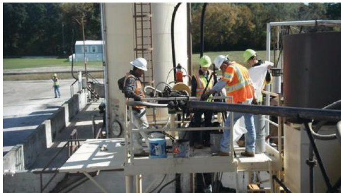
Figure 4-35. Foaming unit on platform, Huntsville, Texas.
