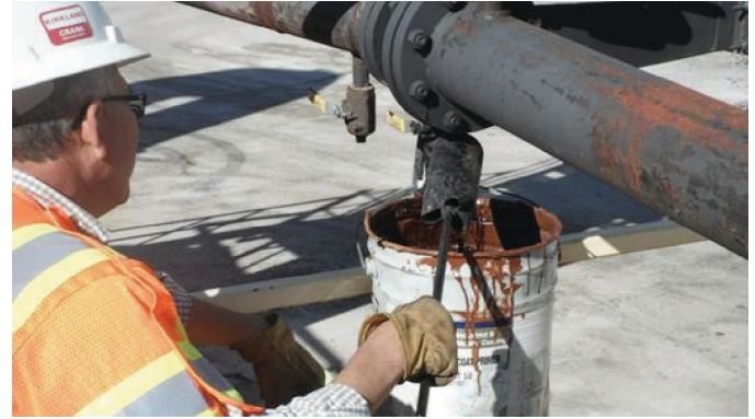
Figure 4-36. Heating valve prior to sampling foam, Huntsville, Texas.
