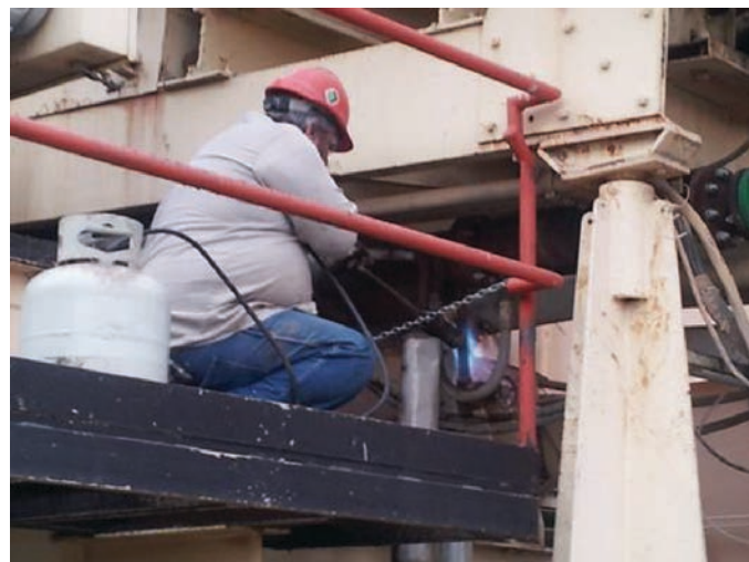
Figure 4-18. Location of foam sampling port and heating to loosen valve, Plant 1, Cincinnati, Ohio.
