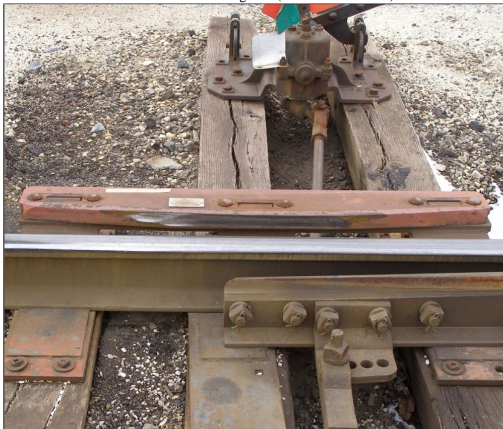
Figure 32. Switch Point Protector
