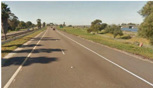
Informal dispersion to median and shoulder, Interstate 8, San Diego urban area (Credit: Google).
