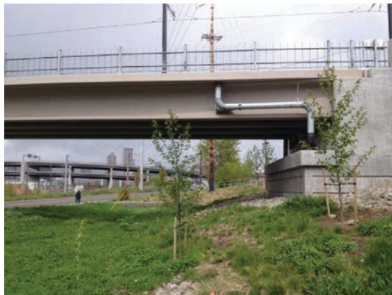
Credit: Geosyntec Consultants Highway 99E Viaduct, Portland, OR.
