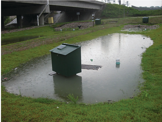
Figure 10. Bioretention cell in North Carolina DOT right-of-way researched by Luell et al. (2011). Source: Stacy Luell, Geosyntec Consultants.
