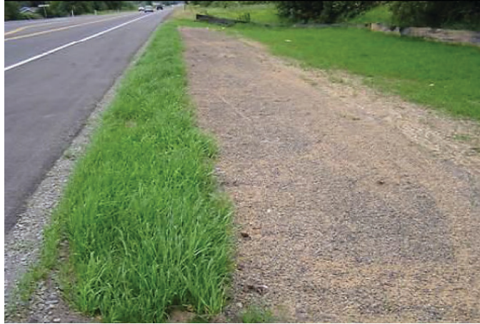
Figure 12. Media filter drain along SR 14 in Clark County, WA. Source: Washington State DOT, 2011.
