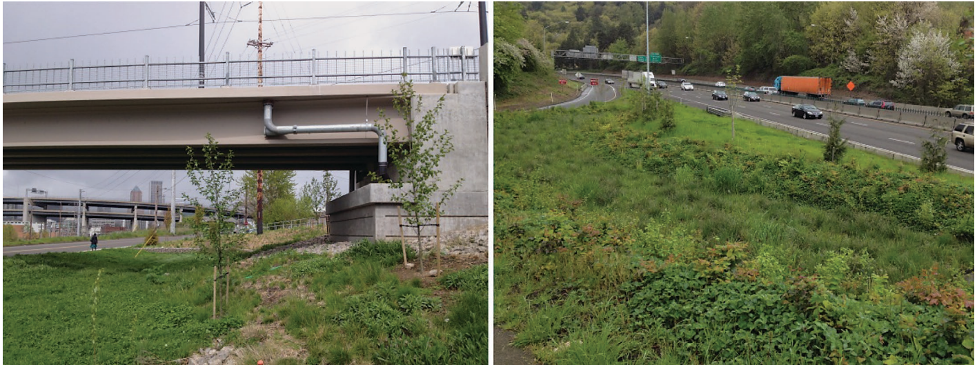
Figure 8. Examples of ODOT bioretention installations. Left: Highway 99E Viaduct, Portland, OR; Right: I-5 Exit 298, Portland, OR. Source: Geosyntec Consultants.
