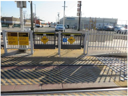
Figure 102. Detectable warning extending on both sides of swing gate.
