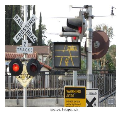
Figure 92. The pictogram within this blank out sign shows a side view of a train approaching from the right.
