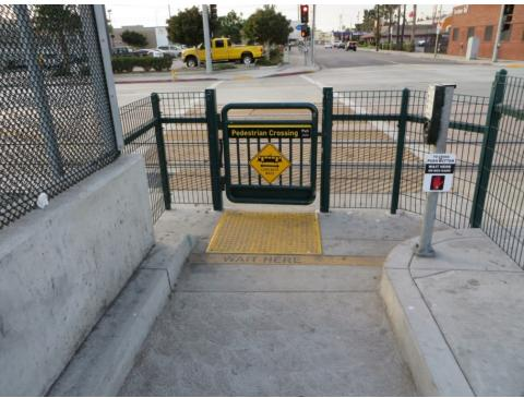
Figure 125. Fencing channelizes pedestrians to crossing location; figure shows well-located APS.
