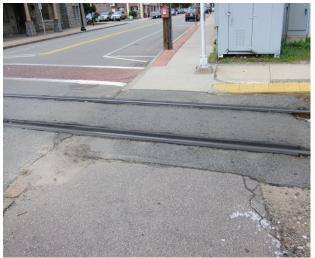
Figure 22. Example of no pavement markings or detectable warnings for pedestrian-rail crossing and solid red bricks within white transverse lines for the nearby pedestrian-roadway crossing.
