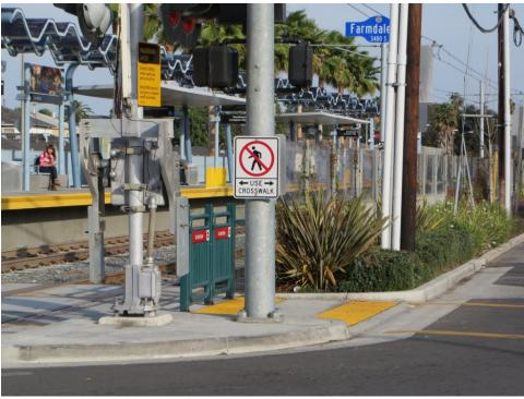
Figure 103. Preferred use of detectable warnings on curb ramp along with swing gate.
