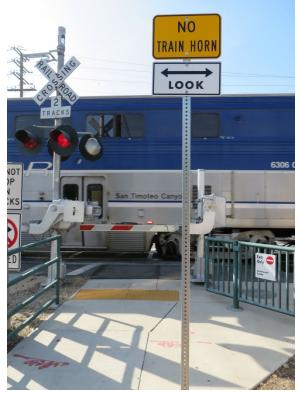
Figure 128. Crossing with automatic pedestrian gate arm with LED flashers at pedestrianonly crossing.
