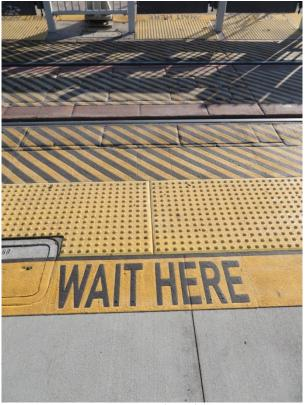
Figure 108. Diagonal striping indicates dynamic envelope of train cars; photo shows location of detectable warning and stop line also.
