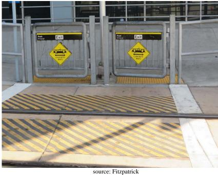
Figure 101. Detectable warning at swing gate on side opposite rails.
