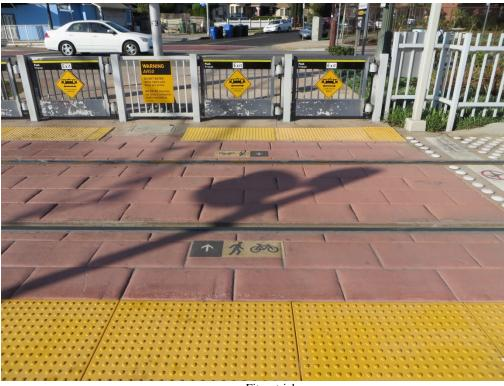
Figure 99. Detectable warning installed inside swing gates.
