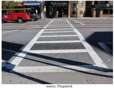
Figure 21. Example of pavement crosswalk markings used with mixed traffic.
