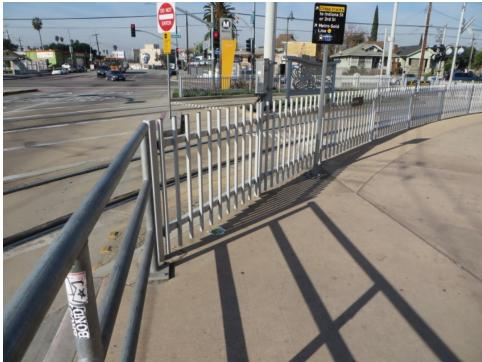
Figure 95. Fencing prevents pedestrians from crossing at the corner and leads to the swing gates at crossing location.
