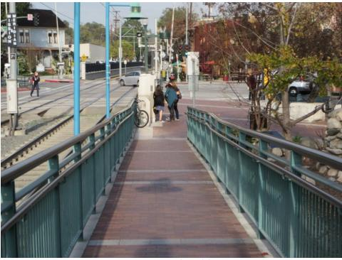
Figure 137. Ramp with attached ADA compliant handrails.
