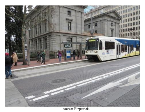
Figure 86. Example of using smooth concrete for train as compared to the brick pattern in neighboring lanes.
