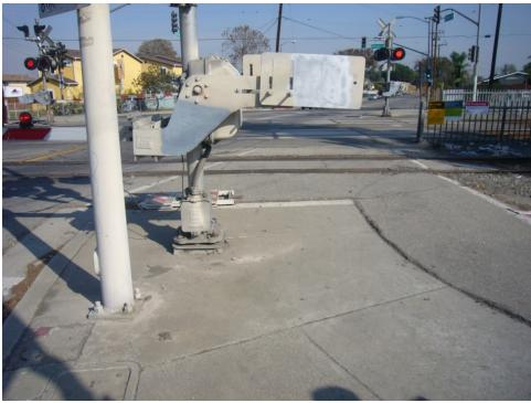
Figure 105. Visually impaired pedestrian has no warning of hazardous counterweight ahead.
