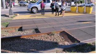
Figure 38. Example of rubber panels providing a distinctive edge of crossing, however, an uneven edge because of the nature of the panels and the angle crossing at this location.
