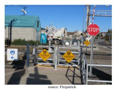
Figure 65. Example of STOP sign with swing gates.
