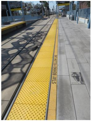
Figure 97. Detectable warning along full length of platform edge with an adjacent yellow line that has STAY BEHIND YELLOW LINE word marking.
