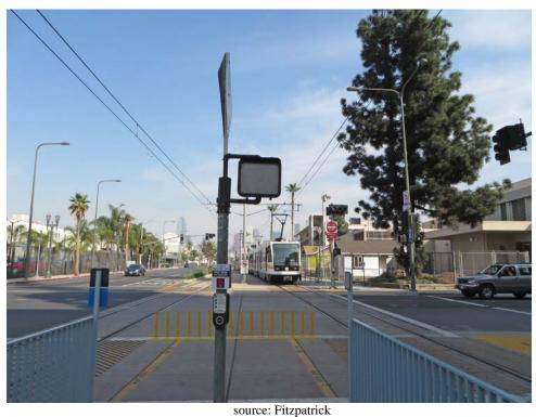
Figure 126. APS at bottom of ramp from platform.
