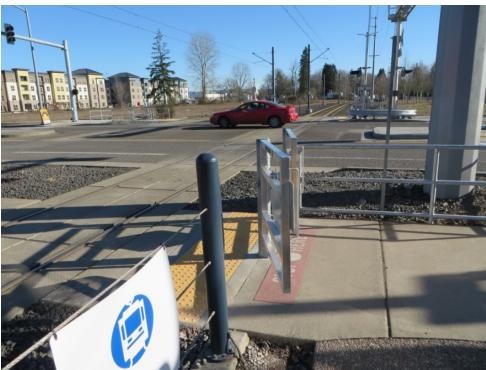
Figure 81. Swing gate being pushed open by wind.
