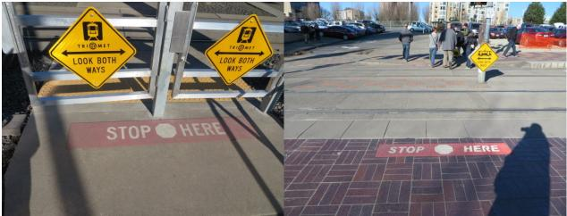
Figure 56. Example of STOP HERE pavement marking in conjunction with a swing gate.
