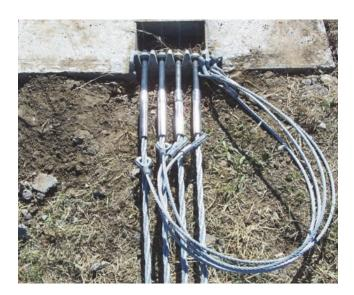
are installed in alignment with the barrier and each cable is attached to the anchor assembly.
