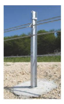
Direct-Driven Line posts can only be used on the TL-3 systems. The post used is 1829 mm (72 in.) long with no soil plate and is driven to a depth of 991 mm (39 in.) into natural *NCHRP Report 350* strong soil. If rock is encountered, follow state's procedure or drill a 4 in. diameter hole to accommodate a minimum of 15 in. of the line post.
