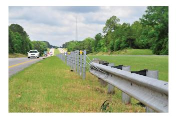
FIGURE 11 HTCB connected directly to w-beam.
