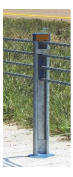
The system configurations using the C-post with a vertical slot at the top of the post are shown below. The direct driven option is shown, but a socketed post design is also available with a 450 mm (17.7 in.) socket and 1230 mm (48 in.) long C-Posts.
