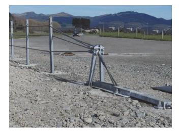
The Nu-Ten End Terminal is a crashworthy terminal and can be placed anywhere within the clear zone. It is used to anchor all the cables to one foundation. It utilizes a trigger post, which will disconnect all the cables upon impact.
