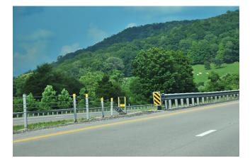
FIGURE 9 Terminating the HTCB in advance of w-beam.
