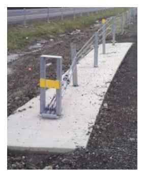
the clear zone. The end anchor consists of an in-ground anchor post, a cable release post and four terminal posts. The end terminal section is 27.5' in length. End anchors should be installed in AASHTO standard soils and be well drained. If soils do not meet these criteria, then soil testing should be done by the DOT or contractor, as per the state's specifications.
