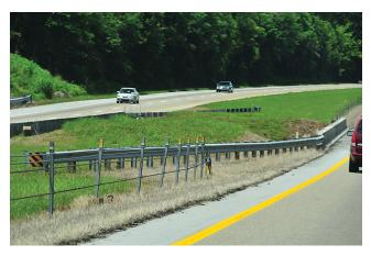
FIGURE 14 HTCB terminated in front of w-beam.
