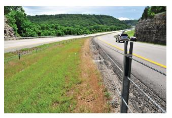
FIGURE 5 Impacted cable on outside of curve.
