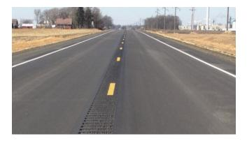
• A **bicycle gap pattern** describes a roadway stretch clear of rumbles (typically between 10 and 12 feet) followed by a series of rumbles (typically from 40 to 60 feet).
