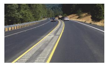
• A center line rumble stripe (example below) is a longitudinal safety feature at or near the center line and created when the center line pavement marking is placed over the center line rumble strip.
