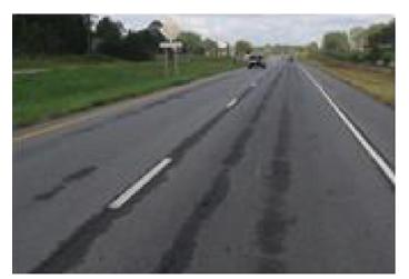
Evidence of moisture intrusion in pavement less than 3 years old
