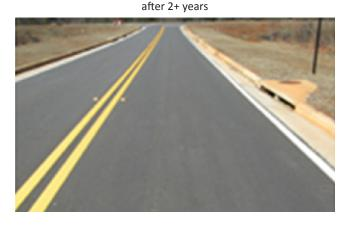
FIGURE 29 Look of high RAP pavements after implementation of the corrected optimum asphalt content (*Source*: Hines 2015).
