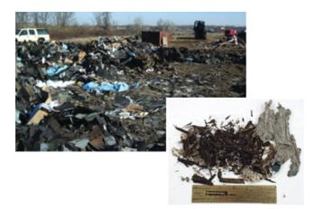
FIGURE 19 RAS stockpiles need to be free of debris prior to grinding (*Source*: Jackson 2012).
